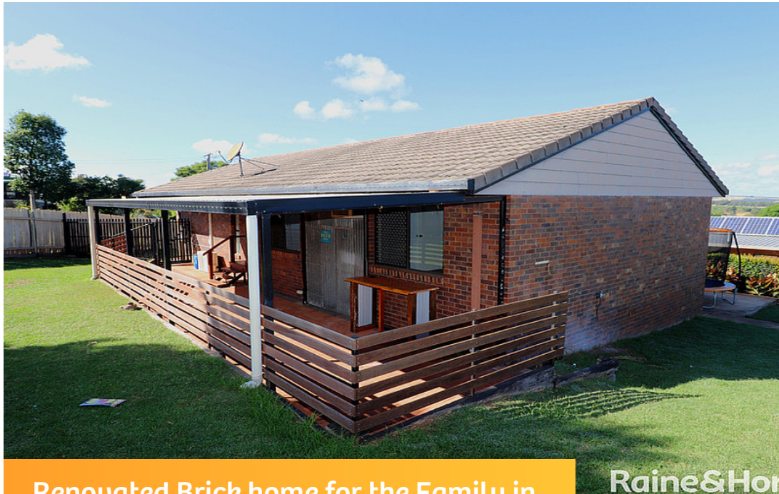
Renovated Brick home for the Family in Sought After Area
