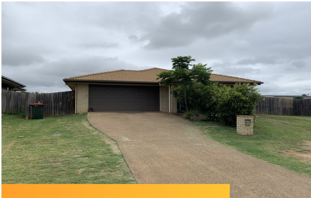
Slightly Elevated Brick House
